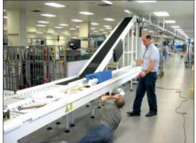
ROLLER & BELT CONVEYOR INSTALLATION. Automatic handling of boxes containing statements for MBNA. This installation uses belt conveyors, roller conveyors and vertical lifters together with gates, escapements and sensors. Controlled by a PLC with a touch screen for operator input.
