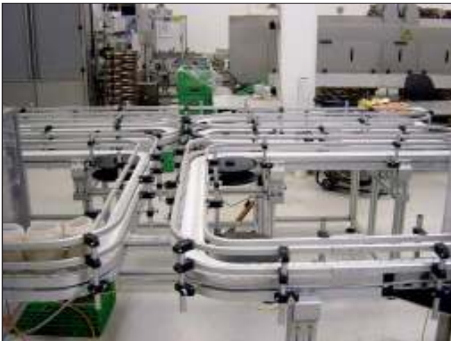
FLEX-CHAIN BUFFER STORE. Typical system handling Horlicks containers in the filling area. This system gives a 20 minute store by the side of the main production line.
