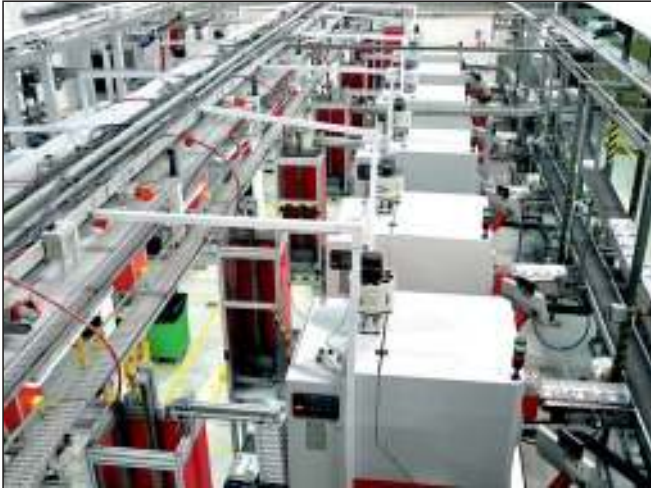
LARGE INSTALLATIONS. Spectacle lens handling plant using our Flex Chain conveyors, flat belt conveyors and vertical lifters. The system handles plastic trays which contain two lenses. A sophisticated but operator friendly control system ensures that trays take the correct path through the plant.
